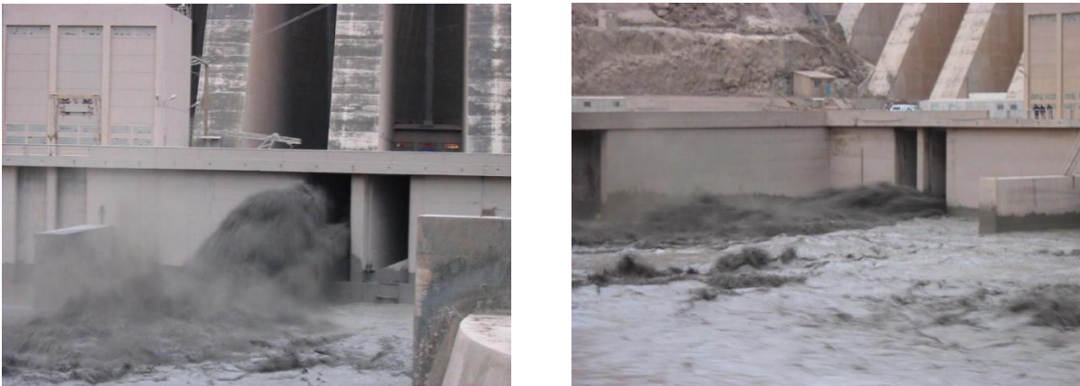
Figure 2.10: Sediment shock load released from Manjil Dam, Iran, during the storage restoration process in 1982-1983, which caused an ecological disaster and a massive extinction of aquatic life downstream.
