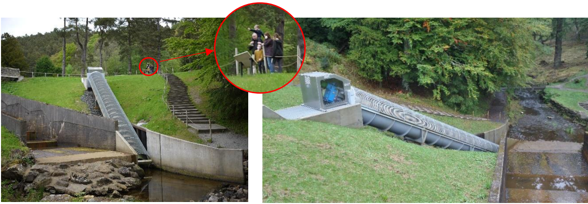
Figure 2.7: Cragside Archimedes Screw Generator (ASG), Northumberland, UK (modified from [87], [88]).
