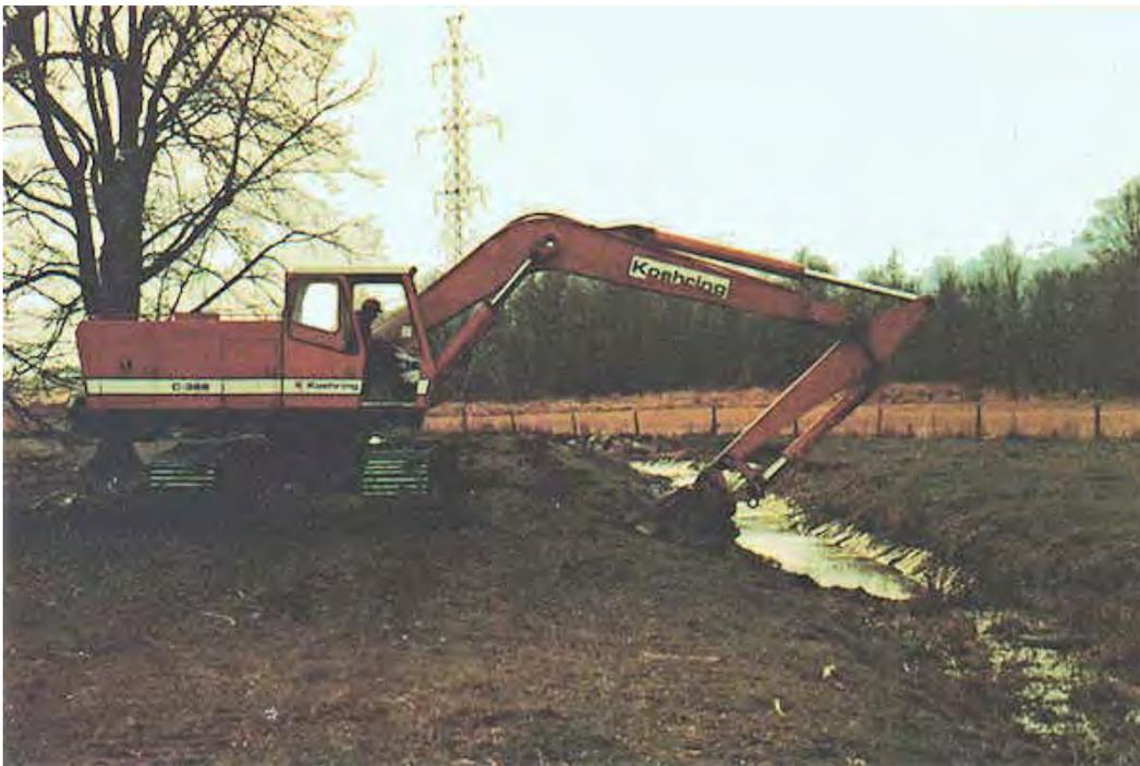
**Figure 10. Regular Drain Maintenance**
